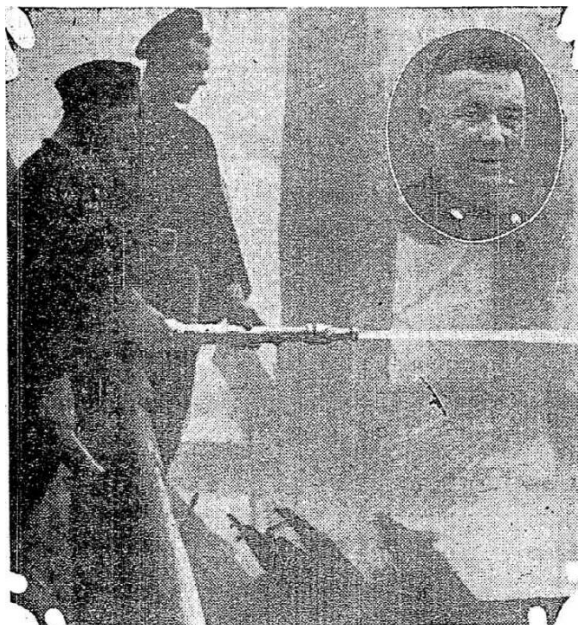
FIREMEN FRASER AND EDWARDS playing water on the smouldering ruins of a two-story building in Bloor Court, City, which was destroyed by fire early this morning. The damage was estimated at £11,500. Inset is Fireman T. Munro, who fell 30 ft. through a skylight while fighting the blaze. He escaped with a severe shaking and several cuts.
