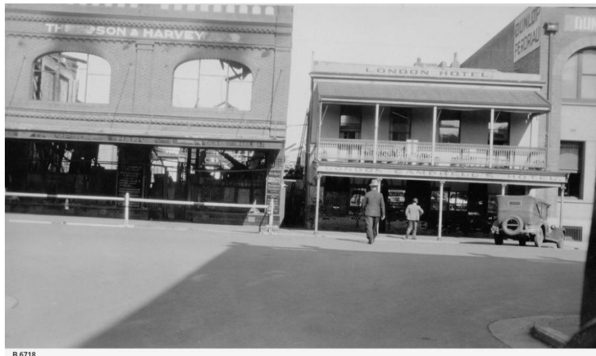
State Library of South Australia - Flinders Street [B 6718]. Flinders Street, south side, 8th May 1935 showing the premises of Thompson & Harvey after a fire. The fire had gutted the premises leaving only the street facade. For photograph of Thompson and Harvey's premises as rebuilt in 1935 see B 6784. Right side is 30 yards east of Roper Street and frontage is 15.5 yards. The London Hotel next door at Number 107 Flinders Street was managed by Miss Annie Maria Campbell from 1919 -1941. 8th May 1935
